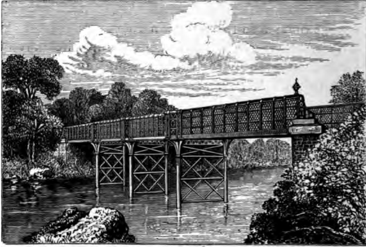
FIG. 72—THE PILMORE BRIDGE.
